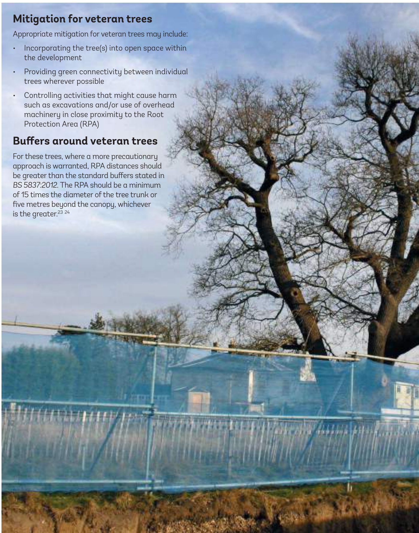
Excavation close to veteran tree
